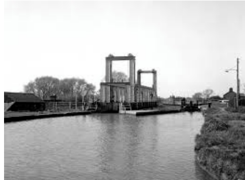
Former steel lock in Rode Heath
